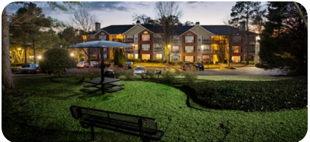
RIVER VISTA 196 UNITS, ATLANTA, GA
